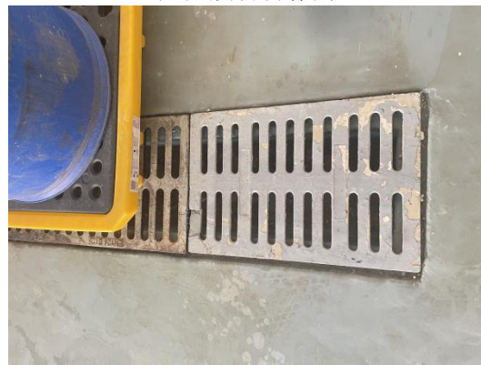
危废仓设无外漏通道的泄漏沟
